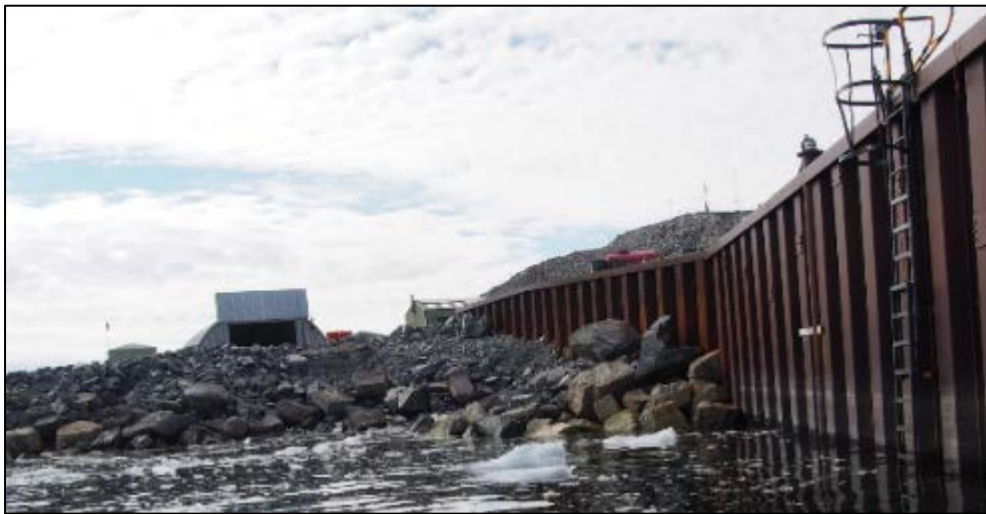
Figure 5-2 Rock revetment in front of the western wall of Biscoe Wharf
