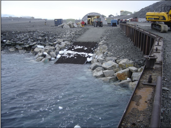
Figure 7-1 Temporary slipway adjacent to existing wharf
