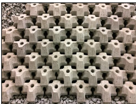
Figure 5-5 Typical X-Bloc Plus Armour Arrangement
