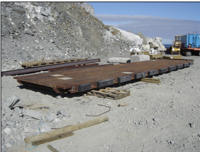
Figure 7-2 Steel slipway prior to deployment
