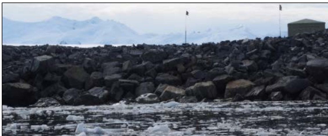
Figure 5-1: Current rock armour across the embankment around the cove
