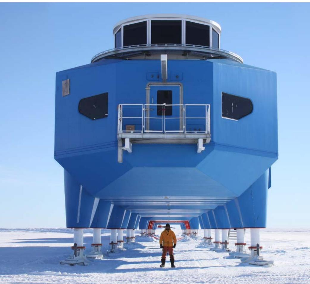
**Image:** Looking along the length of Halley VI Research Station with its hydraulic, ski-fitted legs
